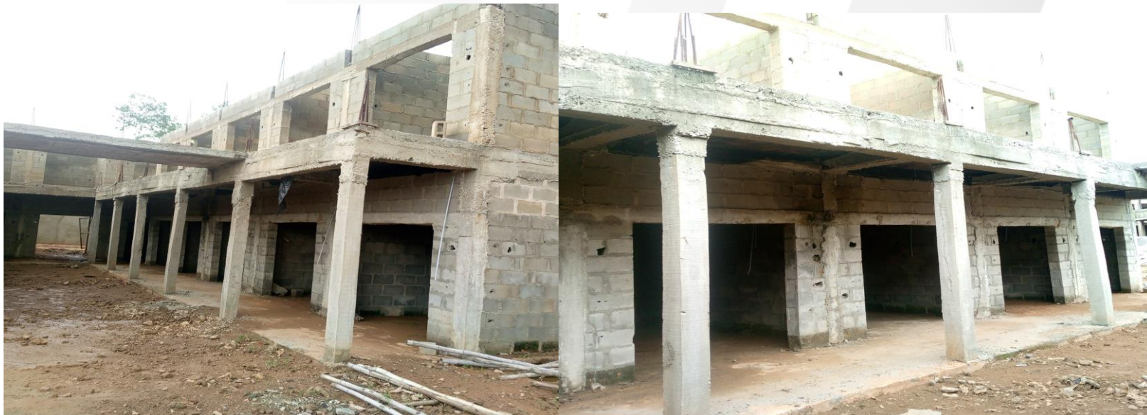
Ongoing project: modern shopping complex at the Aseese Ultra-modern Market in Aseese, Ogun
